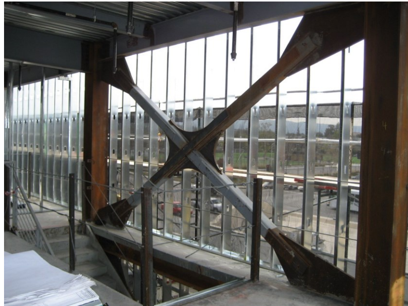
Figure 1-4. SCBF application in three-story steel building in Palo Alto, CA [13].
