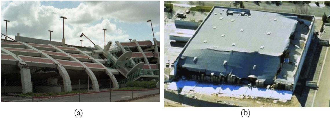
Figure 1-1. Building Collapse During 1994 Northridge Earthquake: (a) Concrete Parking Garages; (b) Storage Building with Rigid Wall Flexible Diaphragm (RWFD).
