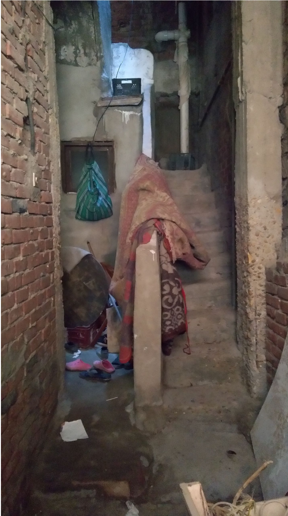
Home entrance in study site 3: Abis slum area
