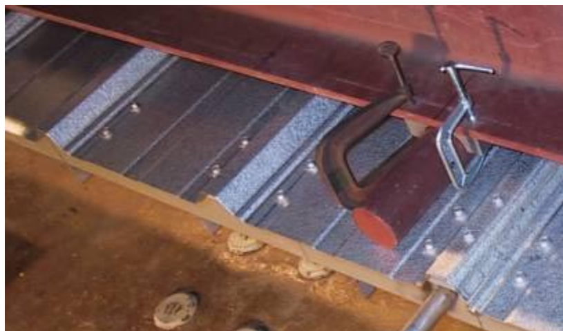
Figure 15 Selected standard panel-to-purlin and panel-to-panel fastener configuration
