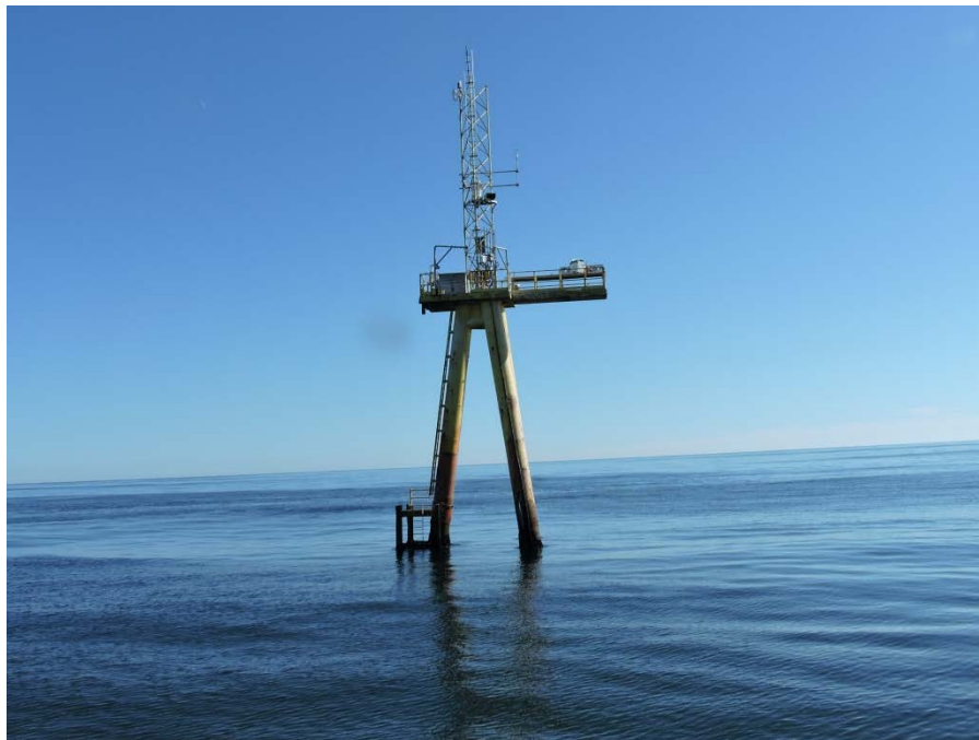
Figure 1: WHOI ASIT Station, View from Northwest – Lidar deployed on the work bench
