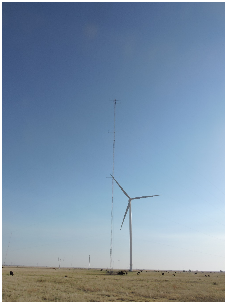
Fig. 3.5 Complete mast overview.
