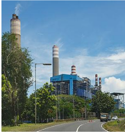
Fig. 4. Steam power plant at PT POMI Paiton
