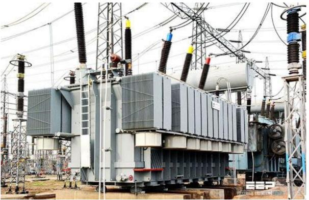
Fig. 1. The power transformer in a substation
