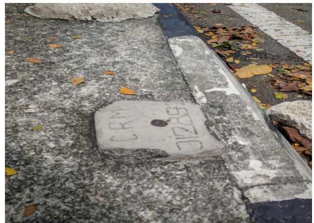
Figure 1 On-site Cadastral Reference Mark (CRM) located beside the road
