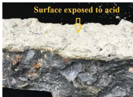
Figure 13. Cross-section of concrete specimen exposed to H_2SO_4 solution.
