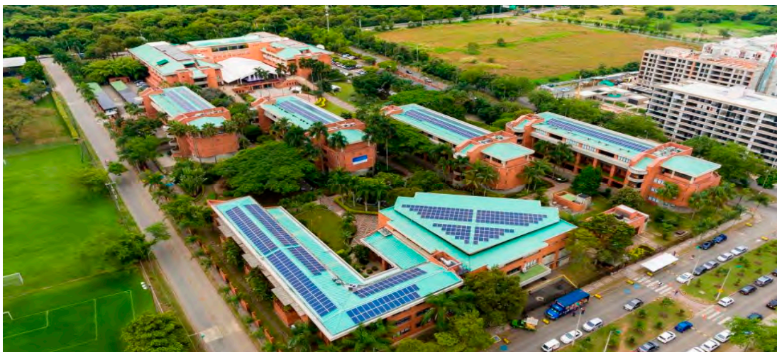
Figure 1. University Campus of the Autónoma of Occidente University (Cali, Colombia).
