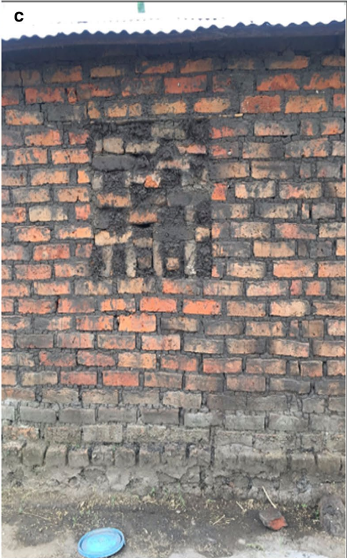
Fig. 1 a An ITN hanging in a rural Tanzanian home. b Screened window. c Eaves and ventilation bricks closed with mud to prevent mosquito entry
