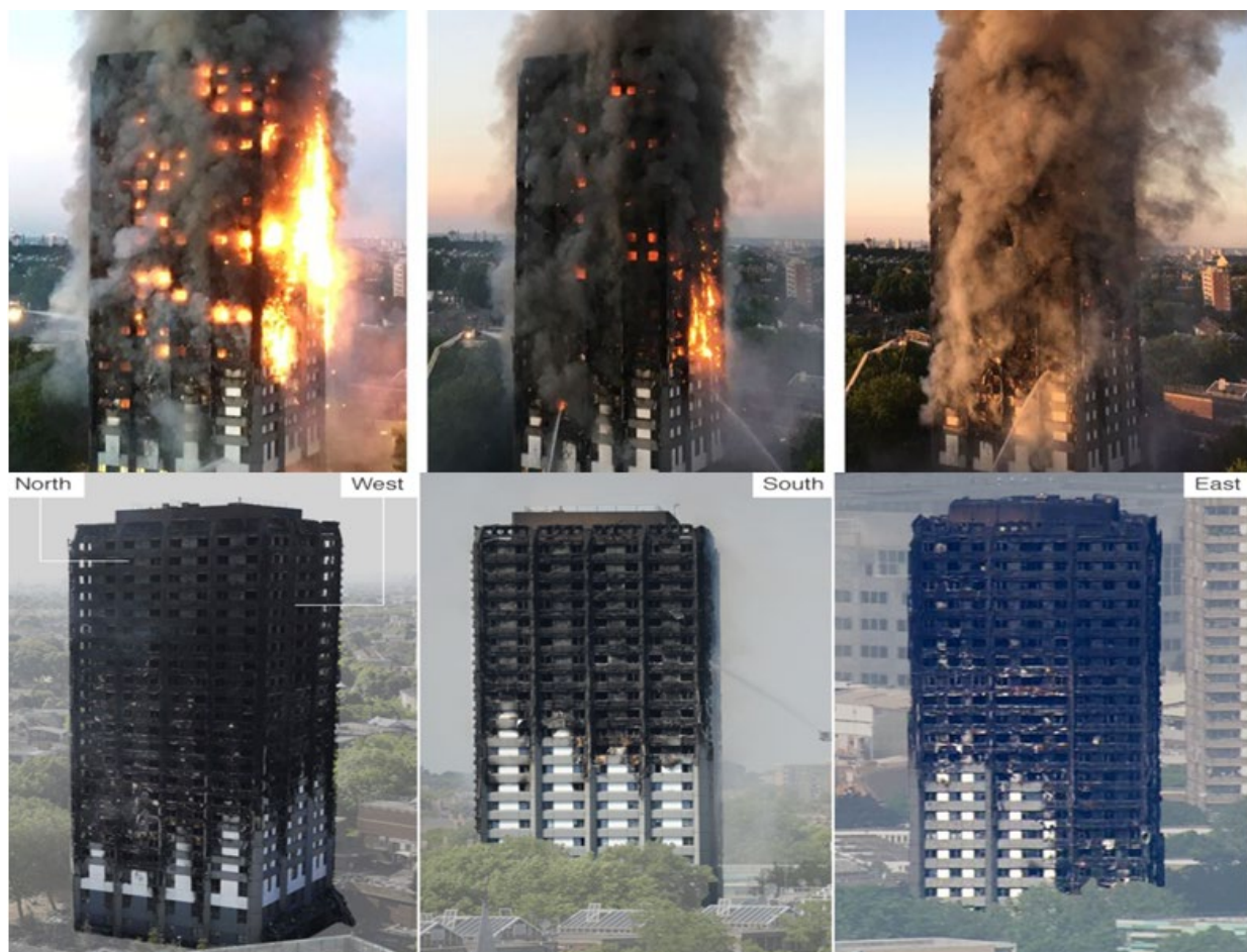
Figure 9. Fire accident in Grenfell Tower, UK [58].
