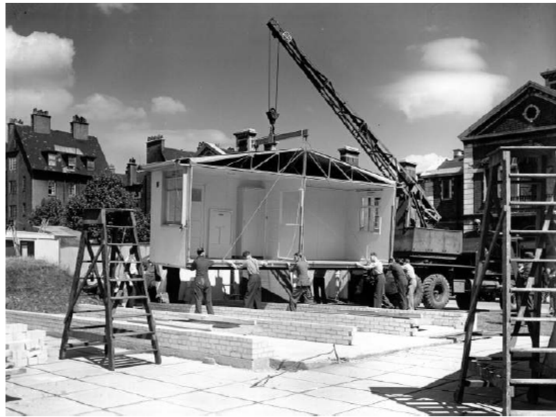
Figure 3. Prefabricated volumetric module at London Exhibition, 1945 [16].
