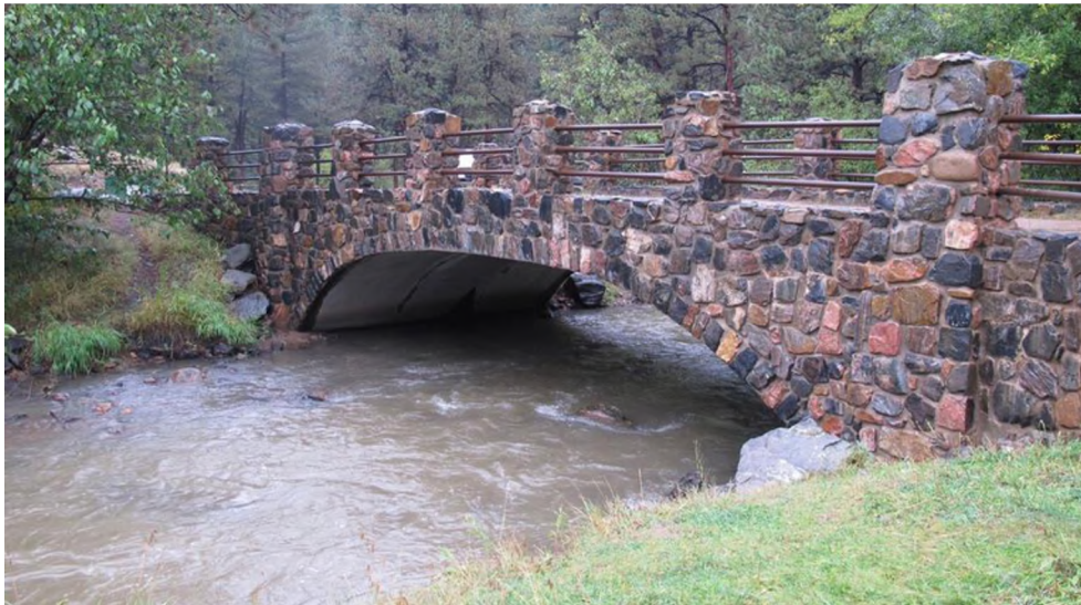
Figure 11. O'Fallon Park Bridge
