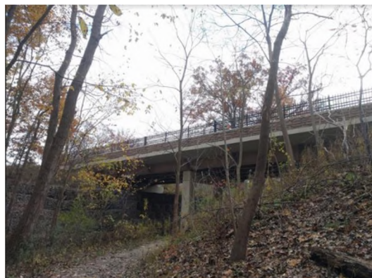
Figure 3. Cuyahoga County Bridge
