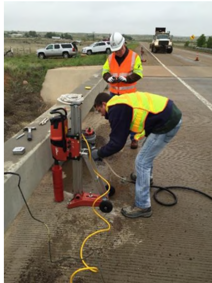
Figure 19. Sierrita de la Cruz Creek Bridge extracted core approximate location
