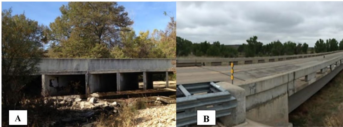
Figure 1. (A) Southview Bridge, Rolla, MO. (B) Sierrita de la Cruz Creek Bridge, Amarillo, TX
