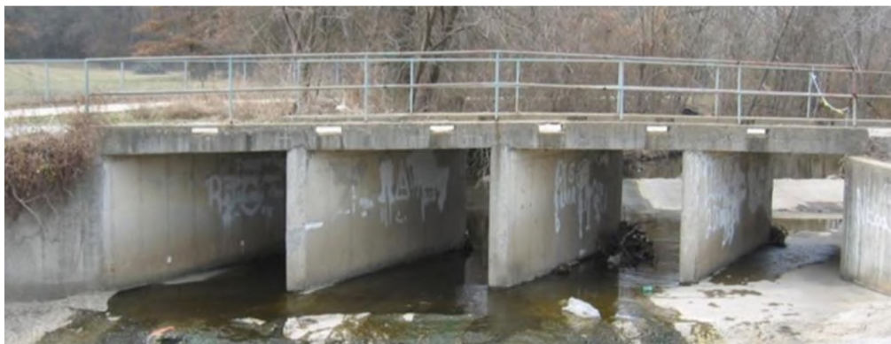
Figure 21. Southview Bridge before extension
