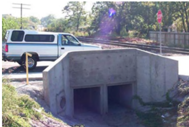
Figure 28. Walker Box Culvert Bridge
