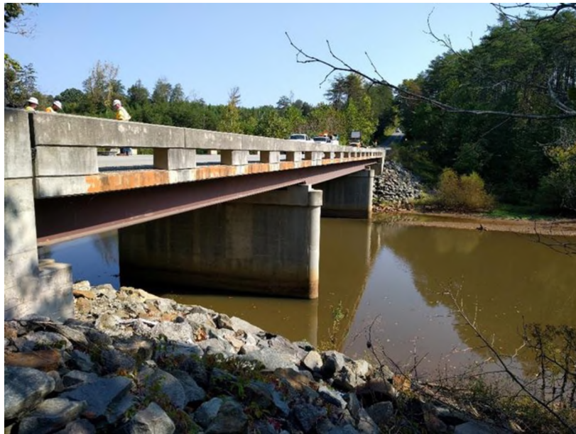
Figure 6. Gills Creek Bridge
