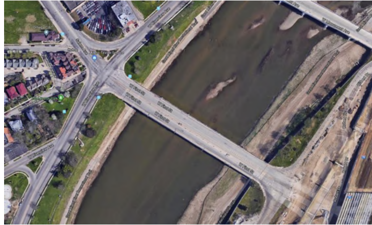
Figure 15. Salem Ave. Bridge aerial view
