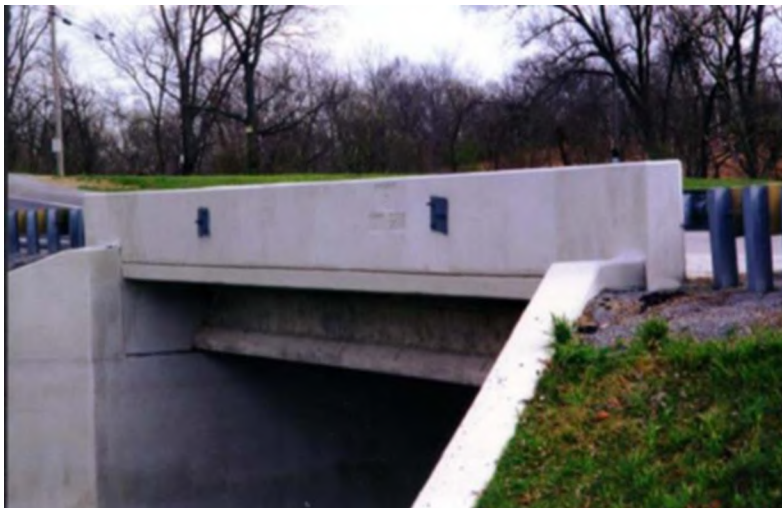
Figure 13. Roger's Creek Bridge
