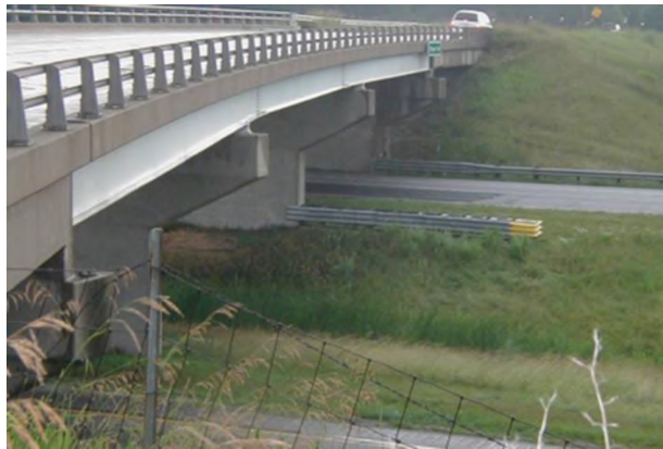
Figure 24 Thayer Road Bridge
