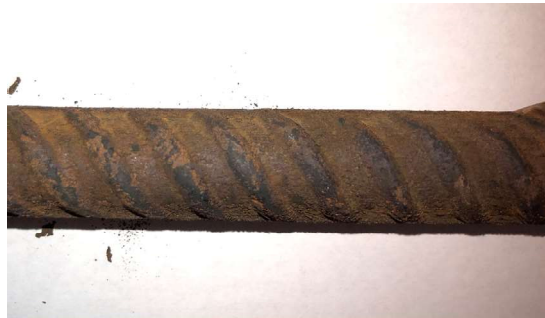
Rebar after corrosion test
