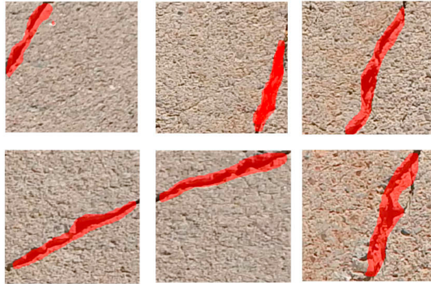
Fig. 4. Examples of detected cracks with the deep learning algorithm
