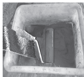
(b) Impregnating and pestling the FRP strips.
