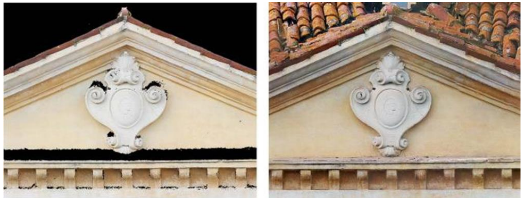
Figure 9. Details of the decoration of the tympanum, on the main façade. On the left the orthophoto obtained from the ground, on the right, the one obtained from UAS
