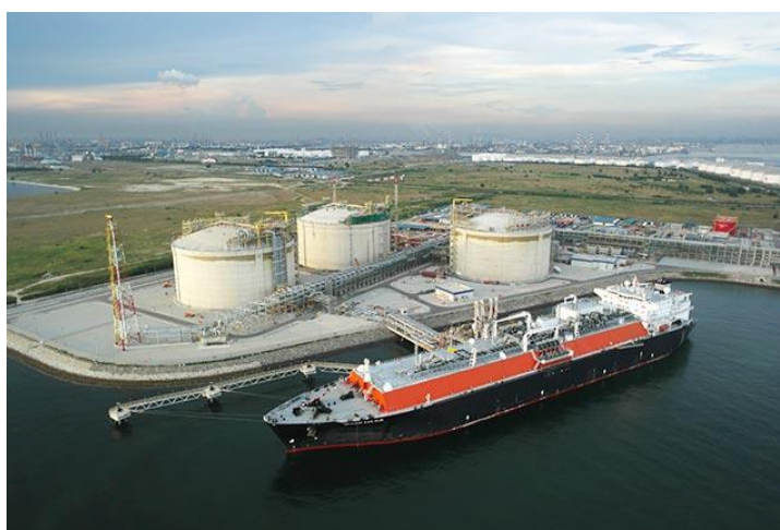
Figure 2.3 Singapore LNG Terminal at Jurong Island in Singapore (Source: http://gcaptain.com/wp-content/uploads/2014/02/02.jpg )
