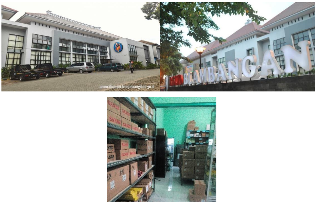
Figure 1.2 Blambangan Banyuwangi Public Hospital and its Pharmaceutical Warehouse. Source: direct capture and Government of Banyuwangi (2017) .
