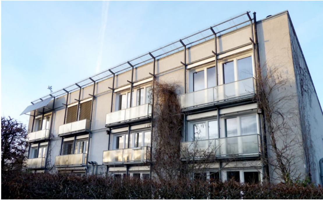
Figure 1-6 The world's first multi-family Passive House, Darmstadt-Kranichstein, Germany 1990 [9].
