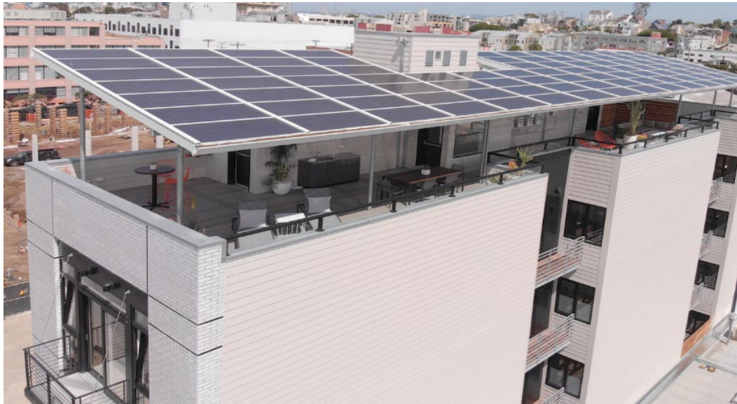
Figure 1-7 Sol Lux Alpha is an energy-efficient building, the winner of PHIUS 2018 [22].
