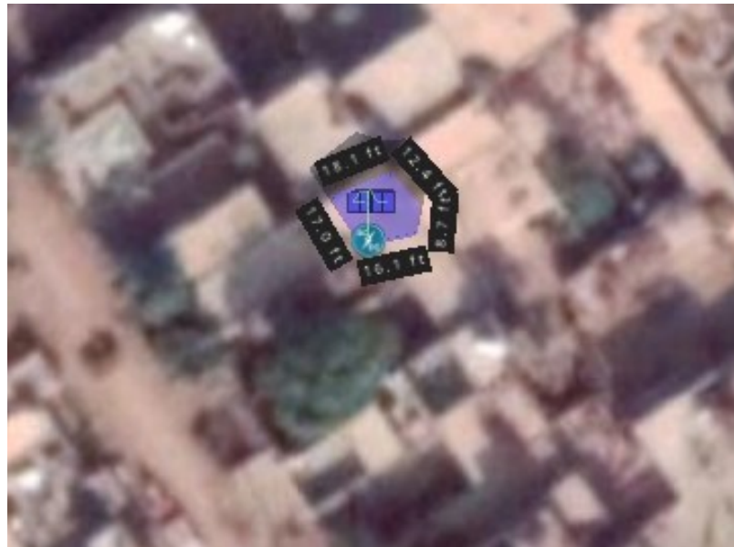
Figure 2.8: Solar panel placement on rooftop
