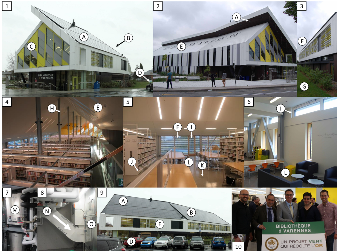
Figure 3.1: Varennes library tagged images. [1] Entrance, south-west view; [2] North facade; [3] South facade; [4] 2nd floor facing West; [5] 2nd floor, middle section, facing South; [6] Ground floor facing South; [7-8] Mechanical room; [9] South facade; [10] Inauguration, from left to right: Dr. Konstantinos (Costa) Kapsis, Dr. Andreas K. Athienitis, Major Martin Damphousse, Vasken Dermardiros and Rémi Dumoulin. (A) Forced convected BIPV and BIPV/T area; (B) Naturally convected BIPV portion (out of view); (C) West facade, vine supports; (D) 2-car charging station; (E) Skylights on northern roof; (F) Fixed exterior louvers, solar shading; (G) Geothermal boreholes; (H) Ceiling fans; (I) Motorized windows; (J) Displacement ventilation integrated to bookshelves/stacks; (K) Underfloor ventilation diffuser; (L) Hydronic radiant slab; (M) Geothermal heat pumps; (N) BIPV/T heat into AHU; (O) AHU.
