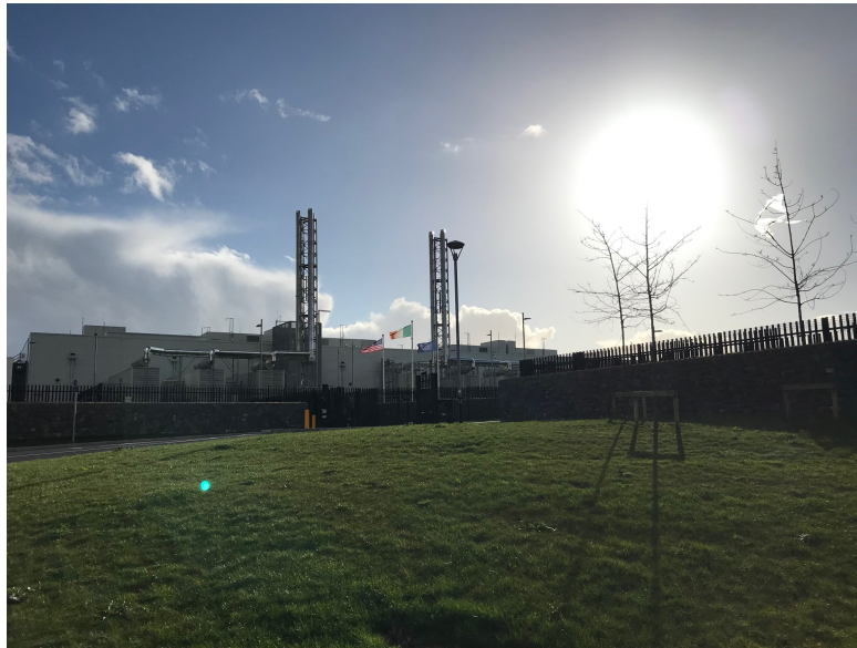
Fig. 50: The securitized gate of Microsoft's Dublin data center campus in Winter 2019
