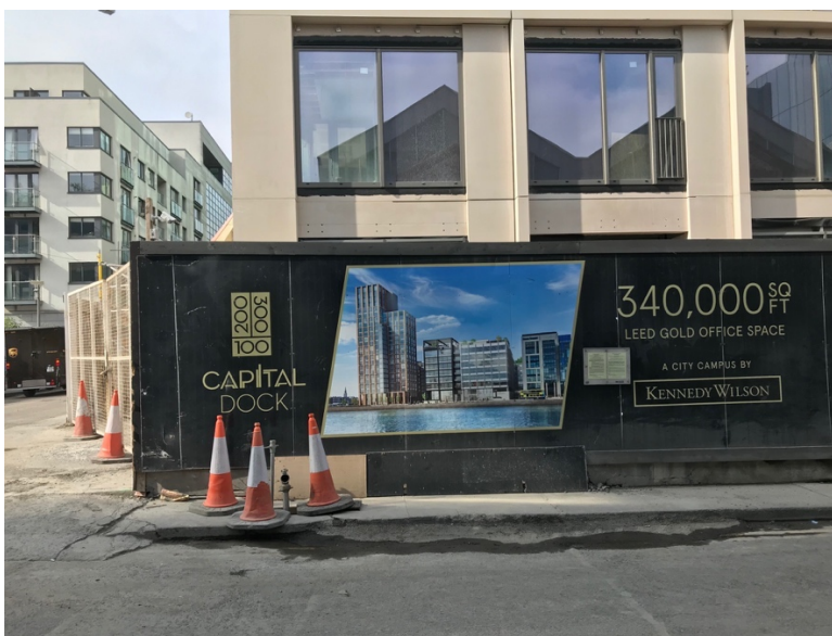
Fig. 9: Construction hoarding around Capital Dock in Summer 2018
