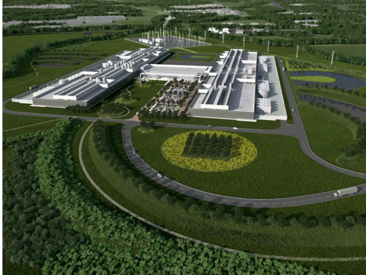
Fig. 55: Digital rendering of Facebook's data center in Clonee, County Meath (source: Sullivan 2016)
