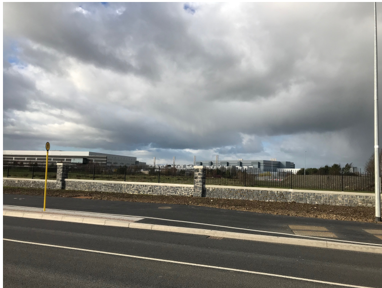
Fig. 56: Microsoft's data center campus in Grange Castle Business Park from a new local road and bike path, Spring 2019
