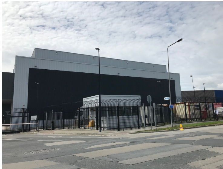
Fig. 48: Faceless AWS data center nearby Tallaght in Spring 2019
