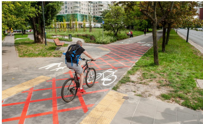
A success story: a surface change in one of the conflict areas
