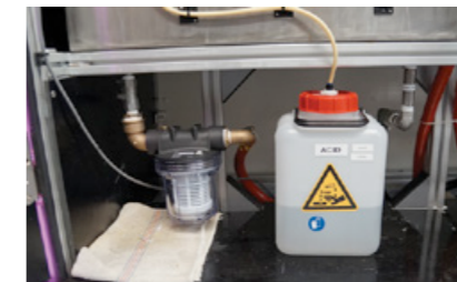
Replaced filter and acid tank underneath the NDS bulk solution tanks
