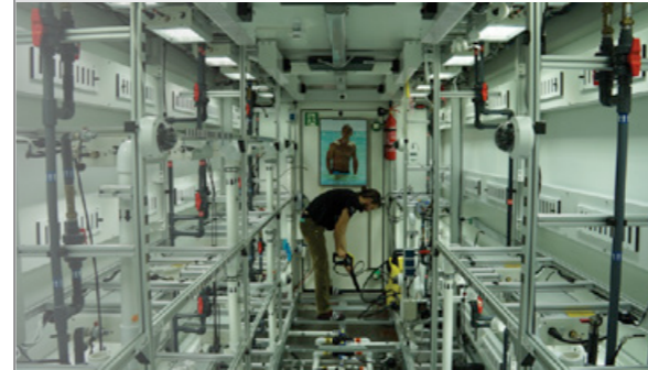
Conrad Zeidler cleaning the FEG subfloor
