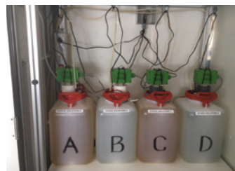
Improved nutrient stock solution tanks were implemented into EDEN ISS
