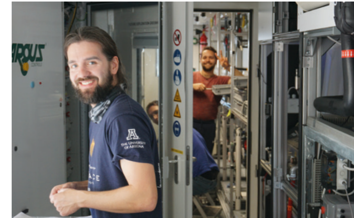
Conrad Zeidler and Markus Dorn installing new sensors
