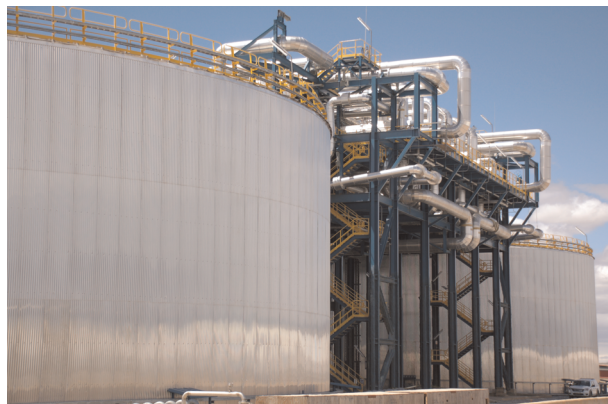
Figure 1. Example of a 1000 MWh th two-tank molten salt storage system of a concentrating solar power plant in Spain (Source: Andasol 3).
