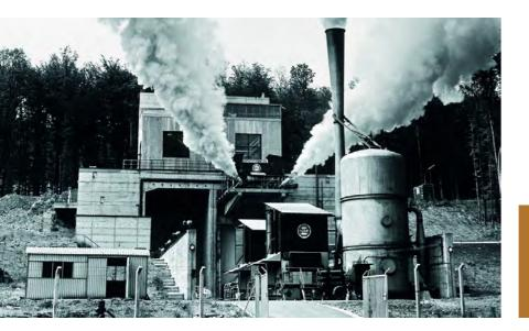
under high-altitude conditions on the P4 test stand. The site engineers developed special steam generators for the operation of the high-altitude system. Since the 1970s, the P4 stand has been retrofitted several times for the Ariane programme. Today, Ariane's Aestus and
