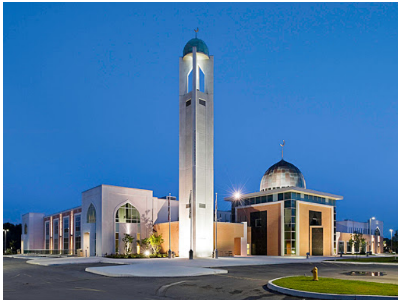
Figure 14: Jaffari Community Centre in Thornhill (Source: Geo Focus Official Website, Accessed February 2018)
