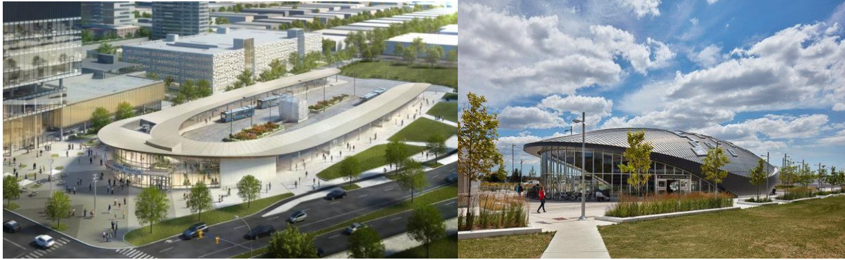
Figure 22 SmartCentres Place bus terminal, City of Vaughan
