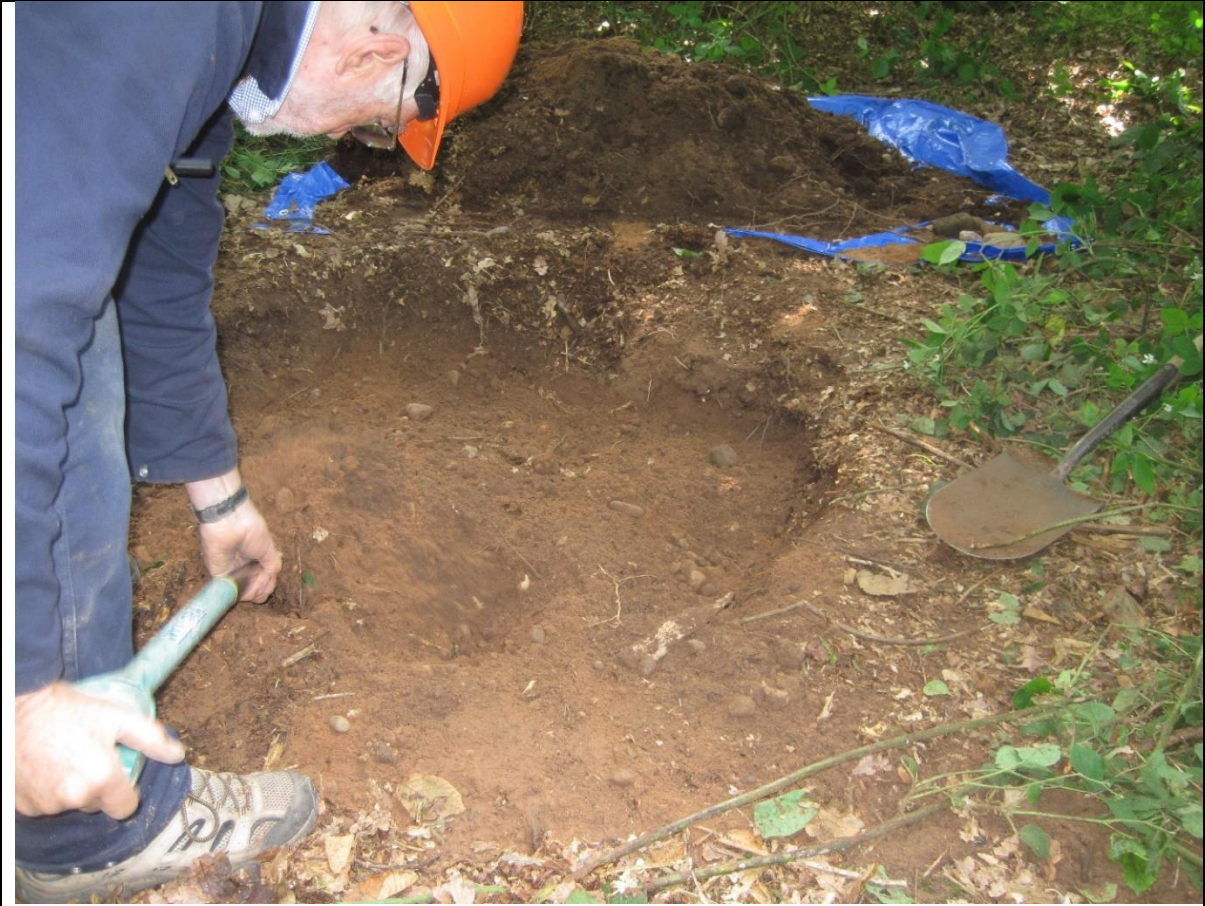
Preparing to replace the topsoil
