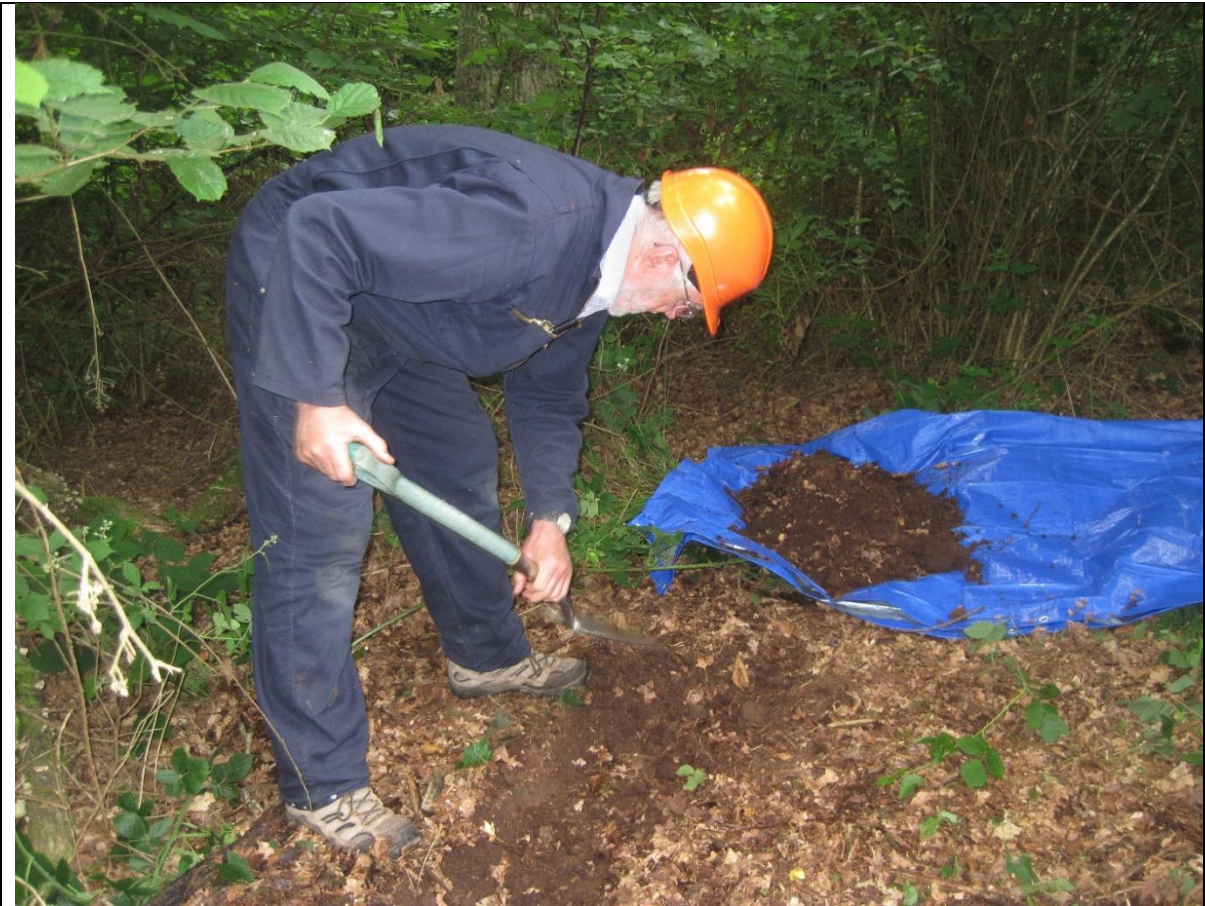
Removing the topsoil
