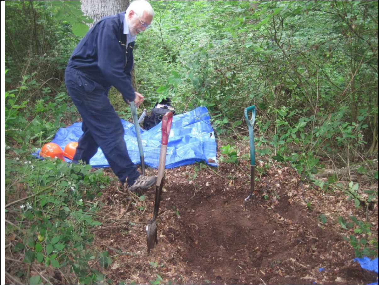
Topsoil removed to a depth of 40cm
