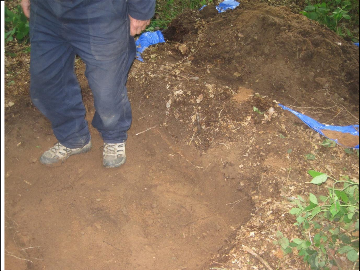
Subsoil returned to the pit, topsoil still in a pile on the side
