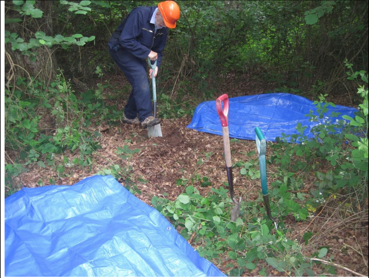
Covering the ground with plastic sheets
