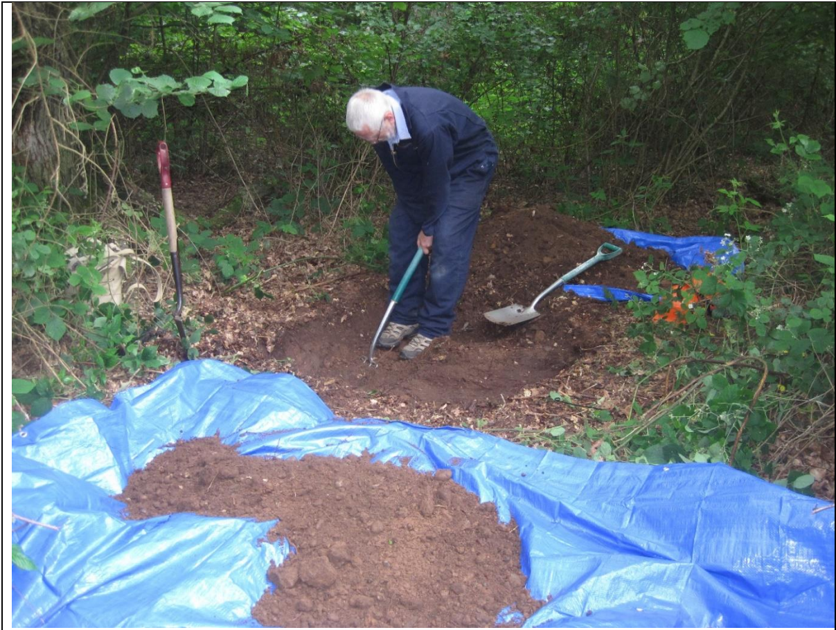
Removing the subsoil below 40cm
