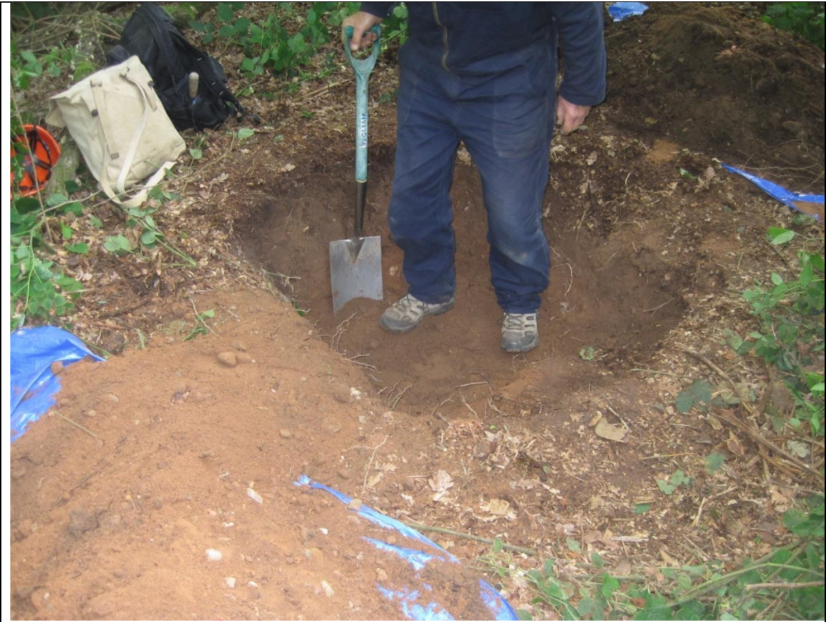
Treading the soil down improve settlement
