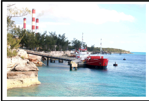
Figure 24. Clifton Pier. View looking southeast toward the docks and other industrial structures along the cliffs today.
