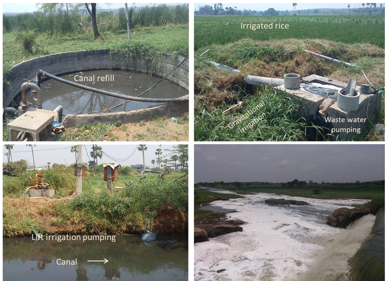
Figure 1.2 Wastewater flows and irrigation infrastructure in the peri-urban node. From top left to right: Wastewater canal refill; Irrigated paddy rice using wastewater from the canal; Lift irrigation pumps from canal to upstream irrigated area; Wastewater attributed flows into the Musi River after the city. Modified from Mahesh et al., 2015a.
