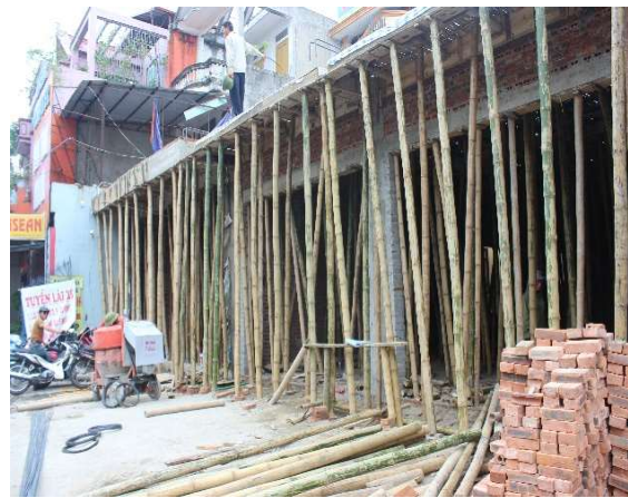
Photo 14. Bamboo poles for construction, Thanh Hoa city
