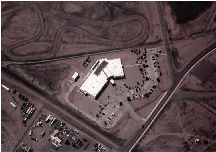
Figure 49: Original Building - Intermediate 1
