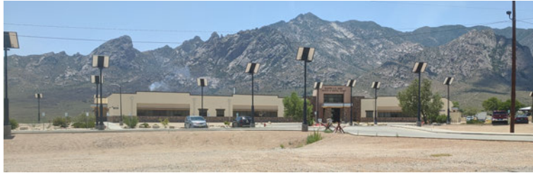
Figure 62: Intermediate 1 Viewed from the Ground
