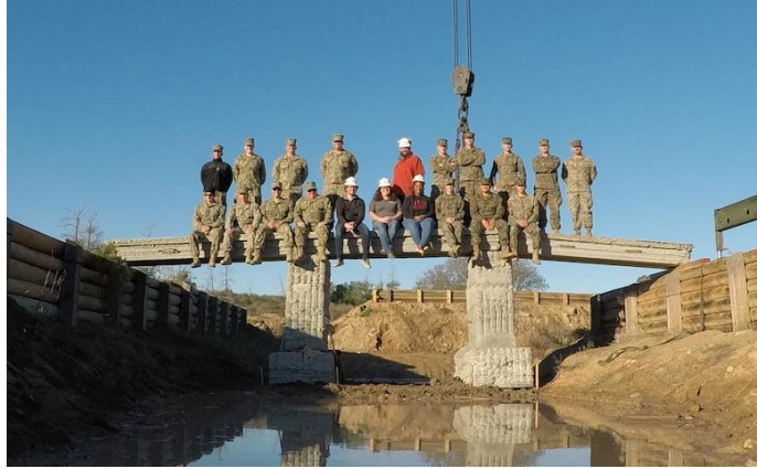
Figure 4. Finished Printed Bridge
