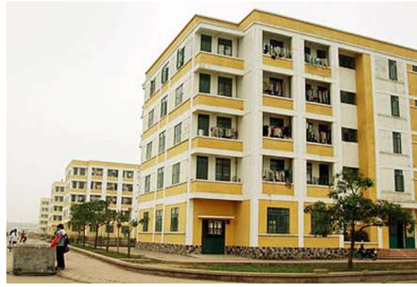
Fig. 6 - Apartment for workers in Bac Thang Long IZ, Dong Anh, Hanoi (Source: Homedy.com, 2017)
