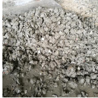
Fig. 8 - Completely Mixed Concrete
