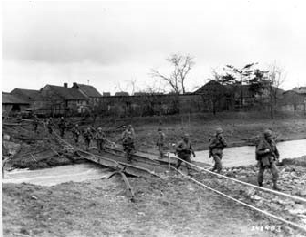
Figure 65 Treadway bridge over the Erft at Bliesheim
