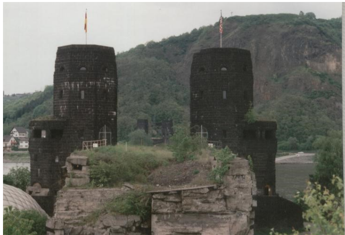
Figure 73 Western Towers of the Bridge - 1990
