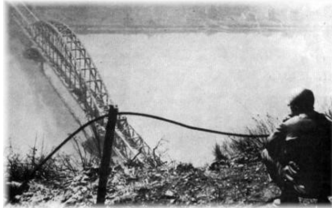
Figure 70 Ludendorff Bridge from the heights above Remagen
