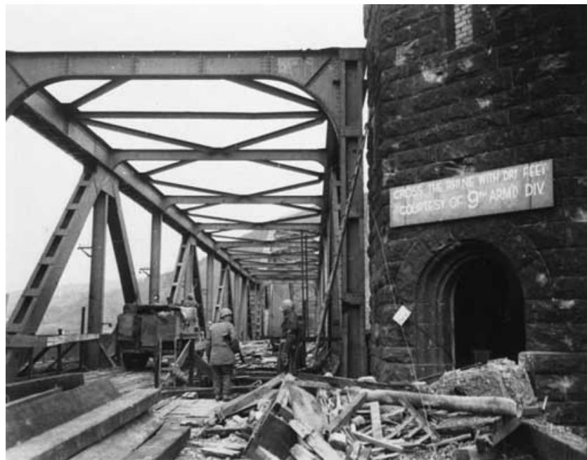
Figure 71 9th Armored Division sign on the Ludendorff bridge March 11, 1945. U.S. Army Signal Corps photograph taken by W. Spangle.
