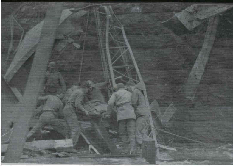
Figure 76 The Bridge collapsed
