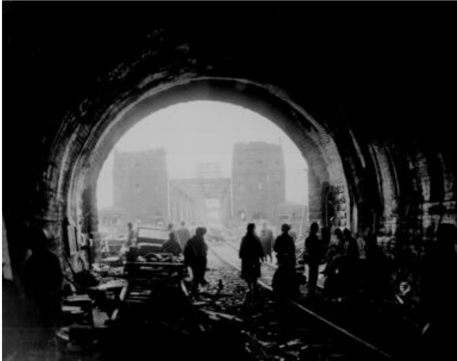
Figure 72 Remagen view from the tunnel
