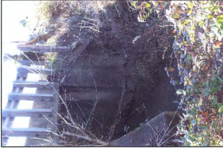
C. An exposed bridge footing at TS01.
