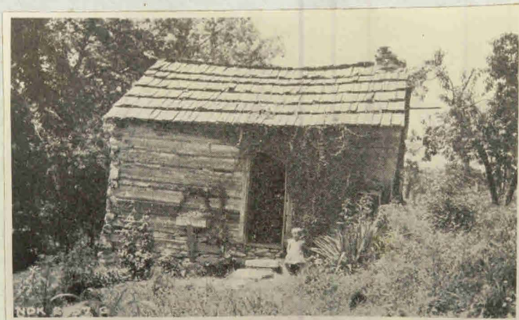
Figure 26. One of the Poorer Homes in the Norris Purchase Area, 1934
