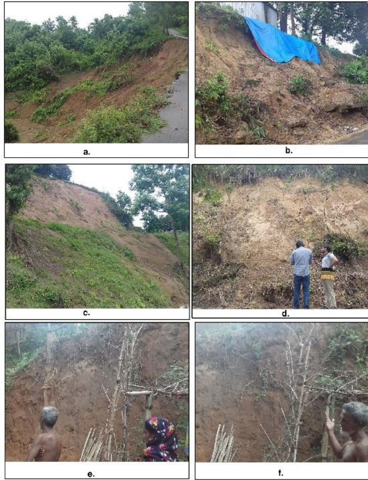
Fig. 2.4. Field Mapping. (a) and (b): Field Mapping with the Assistance of Local People, (c) to (f): Identification of Landslides and GPS Coordinate Collection
