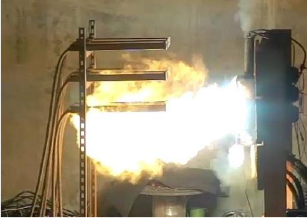
Figure 3 - Arc Flash from a Meter Base
