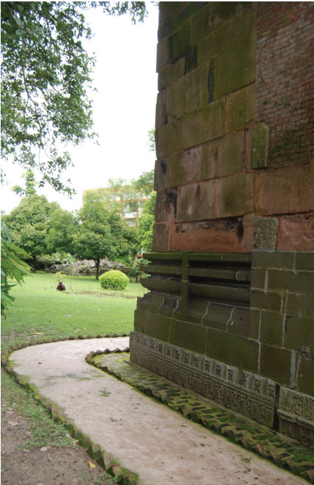
FIGURE 2. Basalt plinth showing the original structure of the building.
