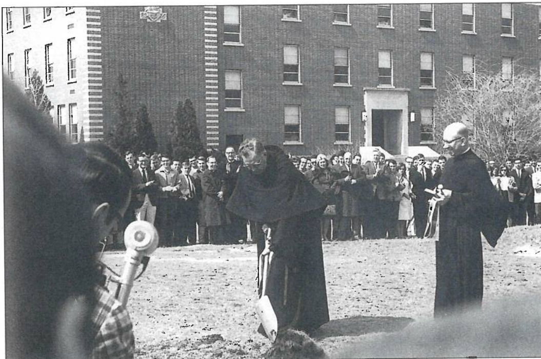
Groundbreaking for the library. Rev. Vincent A. McQuade, OSA breaks ground in the spring of 1966 for the building which later rightly will be named for him as the college's founder. Directly under the left side of the Cushing entrance in the photo is political science professor James J. St. Germain. Just left of St. Germain is Atty. Simeon LeGendre, who taught business law. In the first few years of the college, LeGendre taught in more fields than any other faculty member, including languages and American government courses when necessary, and even aided seniors in placement.
