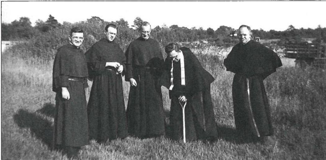
The college operated for two years with only Guild Hall for classrooms, but ground was broken for the science building, the first permanent structure, on Sept. 29, 1948. At the groundbreaking on the former farm south of Elm Street were (left to right) Rev. Francis Smith, OSA, Rev. William J. Wynne, OSA, Rev. Joseph J. Gildea, OSA, Rev. Vincent McQuade, OSA and Rev. James Hannan, OSA. Although it was not completely ready for the college's fifth semester in September, Cushing Hall, which would be the college's science and engineering building until the Mendel Center for Science, Engineering, and Technology, had to be pressed into partial use because of the crowded conditions at Guild Hall in September 1949. Some students had one class in the unfinished new building. In the case of one freshman French class, its odyssey in Cushing began in a first-floor lab in the southwest corner (now the site of Political Science faculty offices) with a very unfinished uneven floor so that every chair tilted (in various directions); that class ended the semester in a third-floor finished lab which was reached by bending down under scaffolding as workmen were setting in the hallway ceiling. Cushing's site is not where the building was supposed to go; it should have been placed approximately where O'Reilly Hall is today as O'Reilly was slated for the present Cushing site, but a site error was made. The building is named for Richard Cardinal Cushing, who had yet to receive the red hat when he pushed for the creation of what became Merrimack.
