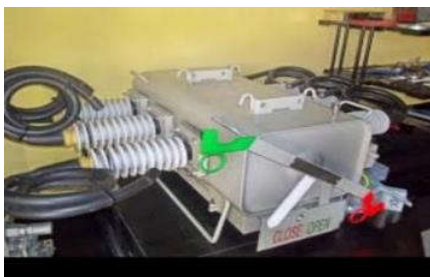
Gambar 2. Load Break Switch (LBS)
