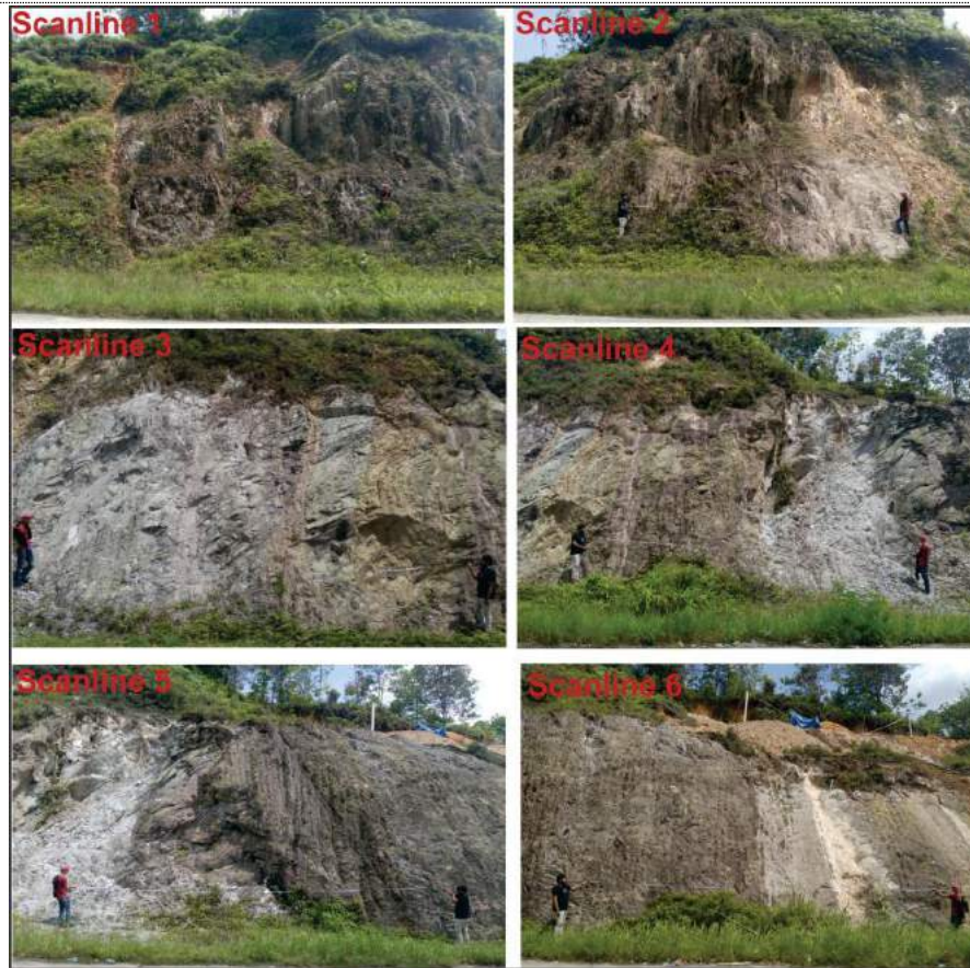
Figure 1: General condition of scanline cut slope
