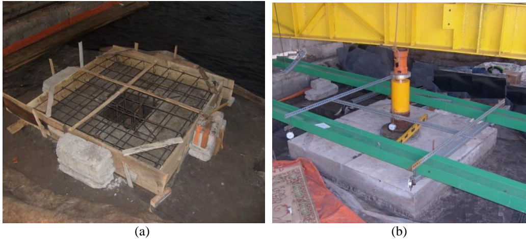
Figure 3 Photographs of investigation on single-pile nailed-slab system: (a) slab reinforcement; (b) loading test
