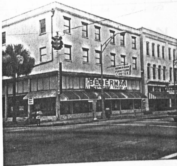
NORTH EAST CORNER 322-328 WEST BROUGHTON STREET 1974
