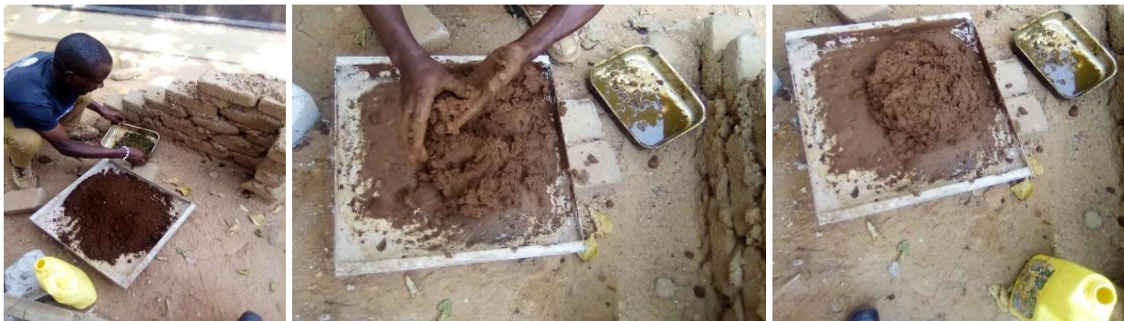
Figure 3: Mixing of cohesive soil with the cow dung
